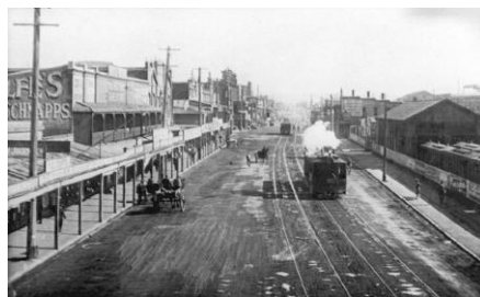
Steam trams in Hunter St passing their shed near Newcastle Station in 1900. Source: Newcastle Herald.
