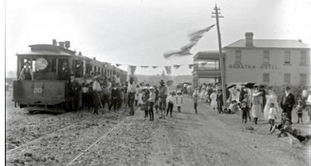
A Mayfield line tram with unsealed right of way. Source: Newcastle Herald.
