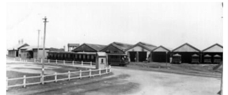
Parnell Place steam tram shed – it was damaged by a shell for Japanese submarine in 1942. Source: Tripod.
