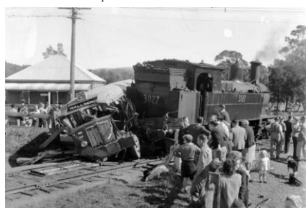
A serious level crossing accident at Toronto. Source: Newcastle Herald.
