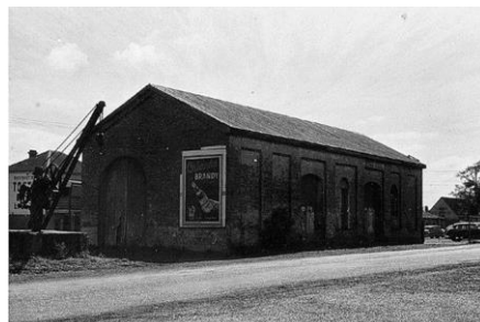
Wallsend Railway Goods Shed in the early Post-WW2 period after line closure. Source: Newcastle Herald .
