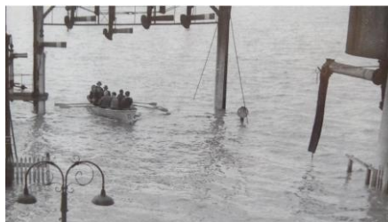
A flood boat being rowed under the Maitland Railway Station signal gantry in 1955. Source: ARHS .
