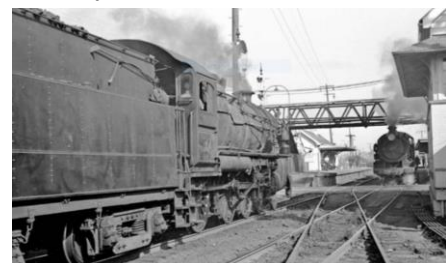
A busy Hamilton Railway Station in the latter days of steam under the watchful eyes in the signal box. Source: Australian Railway History.
