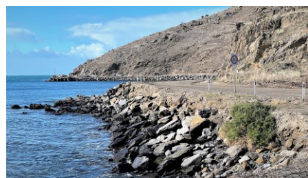
Bluff Jetty Road.
