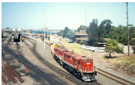
Port Waratah Departure Roads in 1996. Source: David Patterson .
