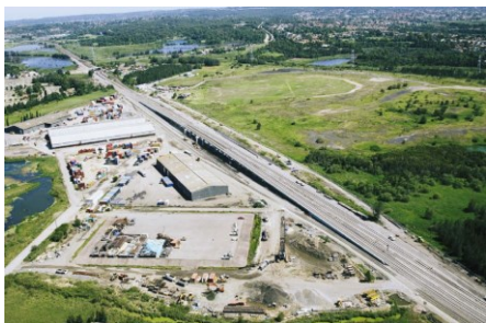
Constructing the 1 in 25 grade 3-kilometre Sandgate Flyover. Source: Arup.
