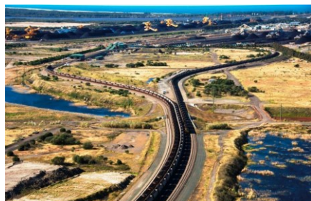
A long train enters a rail balloon loop into a Newcastle coal terminal. Source: ABC.
