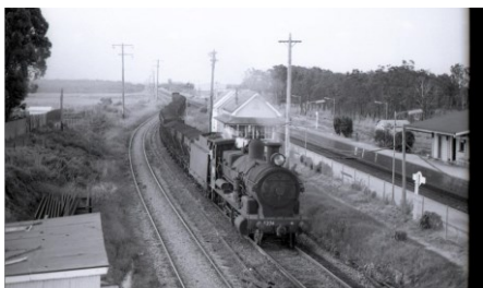
Running the wooden hoppers full of coal to the Port of Newcastle. Source: University of Newcastle.
