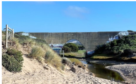
Railway Viaduct over Urimbirra Creek at Watson's Gap.
